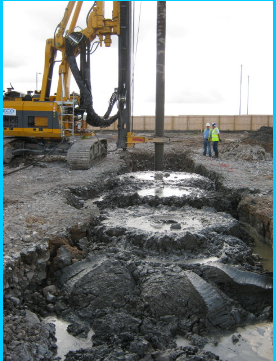
2.0m diameter SM Columns 20m deep
