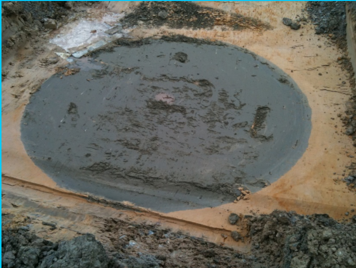
2.0m diameter SM Columns 20m deep
